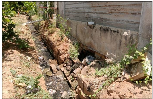
Discharging Waste water – near MM Plastic Industries
