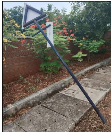
Signage board damaged – near diamond bucket industry
