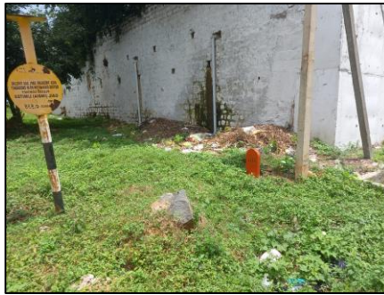
Sewage dump- near KPTCL side
