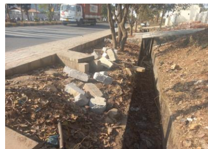
Construction materials dump near M/s SS food
