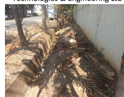
Waste dump near M/s Pasolite Electricals Pvt Ltd
