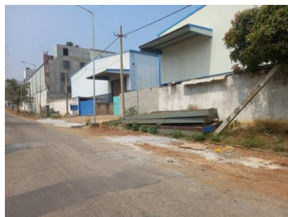
Construction materials dump near M/s Gean Electronics Pvt Ltd
