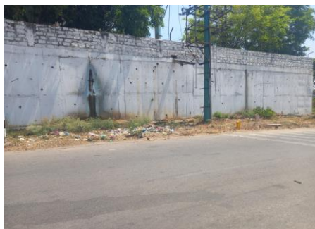
Waste dump near M/s Rajhans Enterprises
