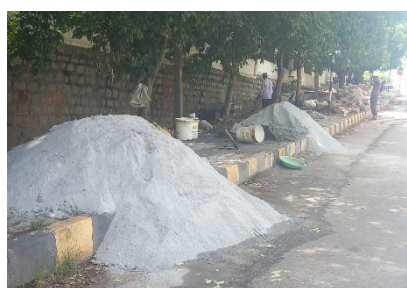
Waste dump near M/s Mahendra industries
