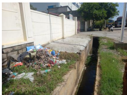
Waste dump near M/s Ambika Sales Corporation
